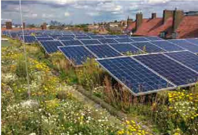
Green Roof Solar
